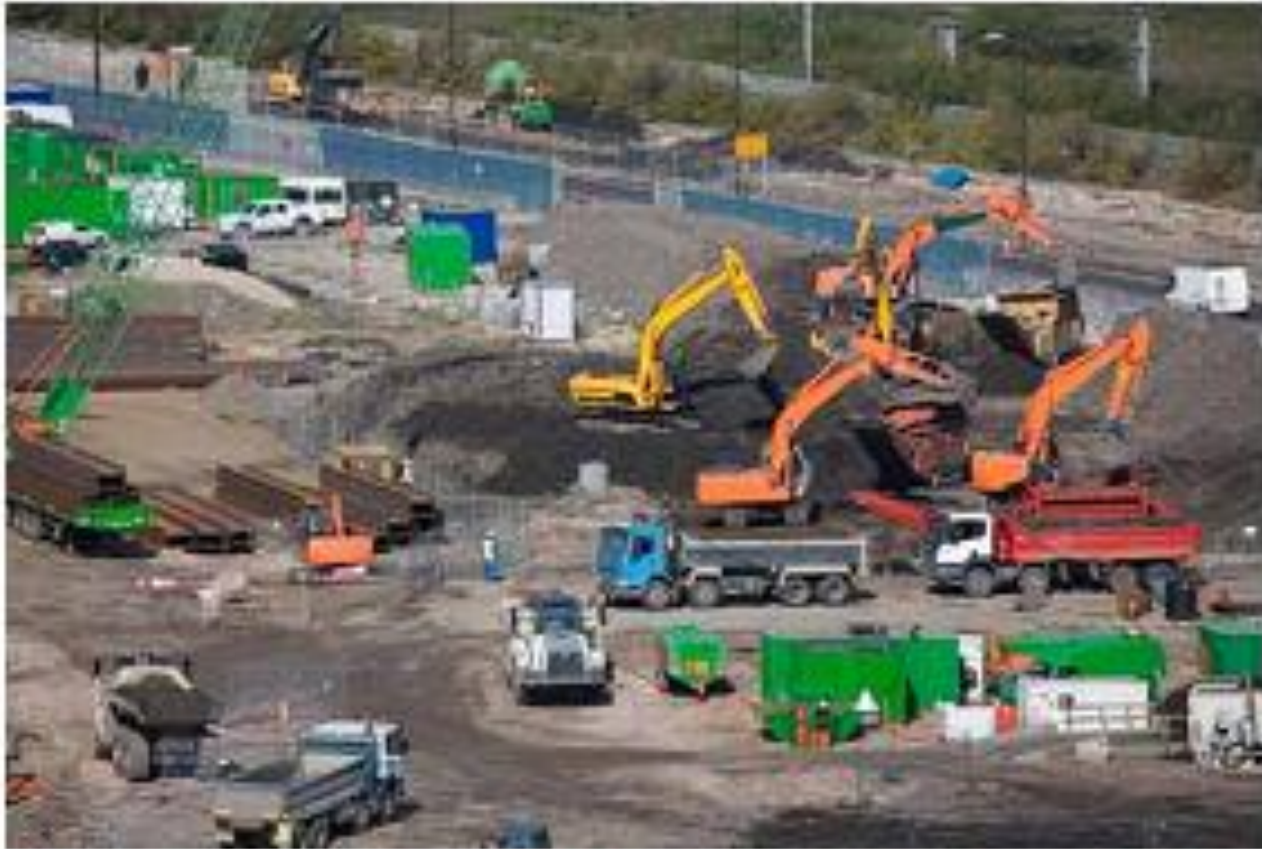
The removal of contaminated soil from the Aquatics Centre site, September 2007
