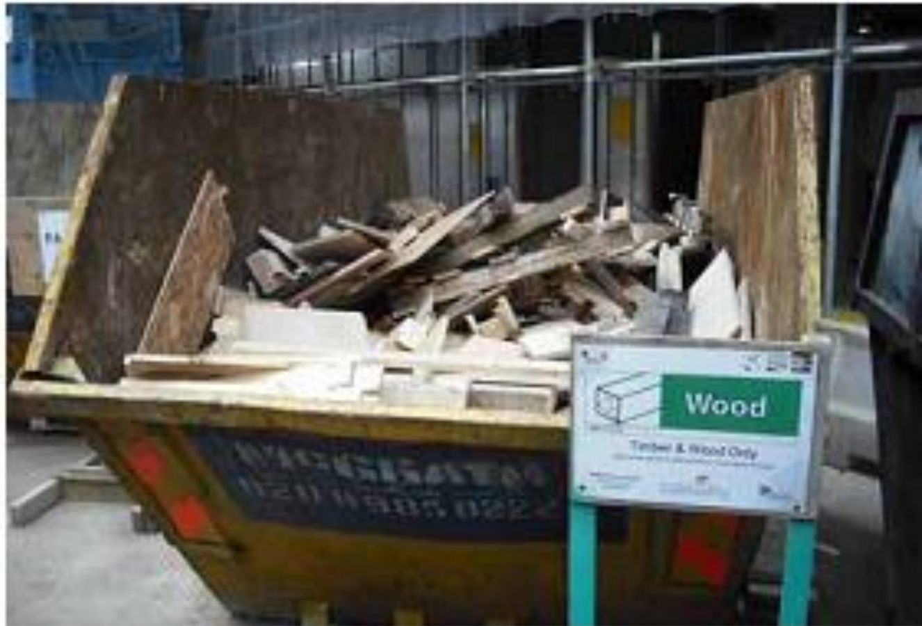
Segregation of construction waste
