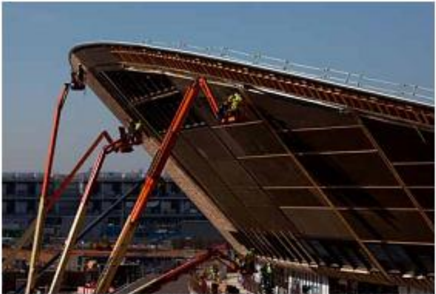
Construction workers applying external cladding to the Velodrome, October 2010
